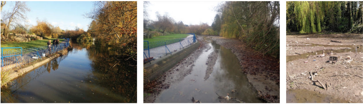
Figure 1. The first photo taken of Osbaldwick beck from a bridge at the lower reach of the beck in Hull Road park before the river restoration works had begun, demonstrating how the beck had been transformed into a series of ponds. The second photo was taken in the same place shortly after the Environment Agency had carried out the engineering works to partially remove the lower weir which drained the beck revealing the build-up of silt. The third photo was taken in the middle reach of the beck in Hull Road Park demonstrating the litter and debris revealed in the silt left behind once the water levels had continued to decrease.
